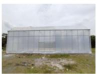
The kit comes complete with everything you need, including steel framework that has been hot galvanised and zinc coated, high quality greenhouse film, wiggle wire and channel, and all the connectors. No welding is required. There are two sliding doors, one at each end of the structure and the side panels that can be opened for better ventilation.
